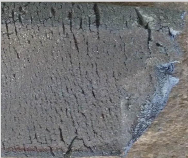
Figure 1. Overheated material with its characteristic cracks from the edges towards the center of the piece.
